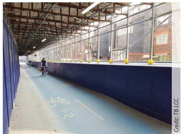
A cycle tunnel has been used here to avoid diversions and the need for cyclists to dismount
